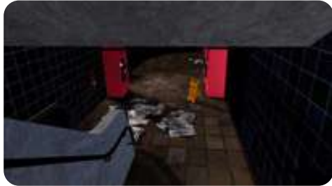
1. Darkness in a pedestrian underpass
