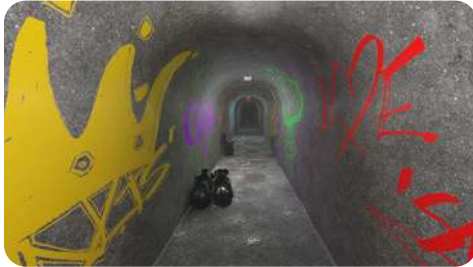
1. Dirty underpass with unsanitary conditions
